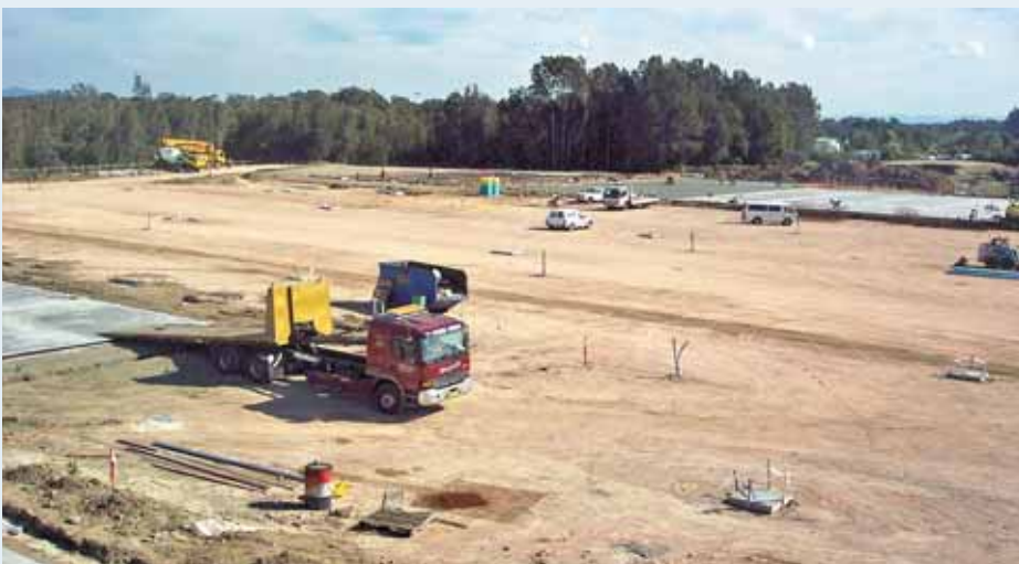
The Port Macquarie, NSW, Port Home Zone construction site.
